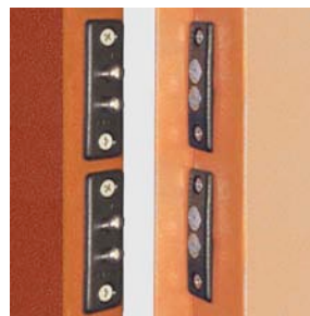
Double electrical contacts between leaf and doorframe
