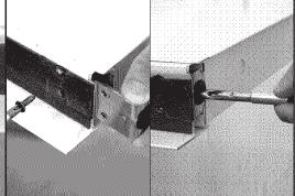
Screw the internal, lower guiding angle by the selftapping screw and insert the rod.
